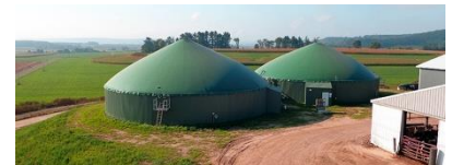
Fig 7: Farm AD concrete tank
